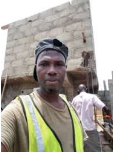
Training center construction
