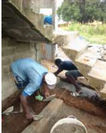
Staircase construction
