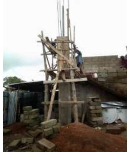
Concrete pillar construction
