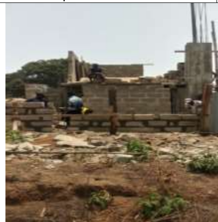
4 room extension block work
